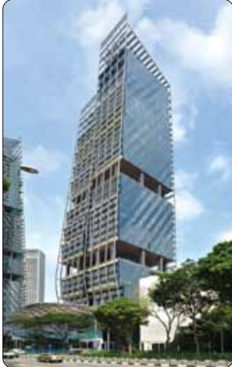
South Beach Tower 46,000 m 2
