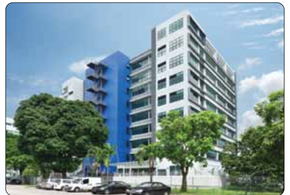
Data Centre at Paya Lebar 3,500 m 2
