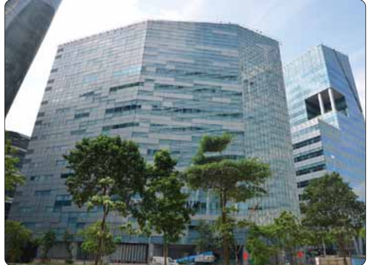
Fusionopolis Development Phase 5 52,000 m 2
