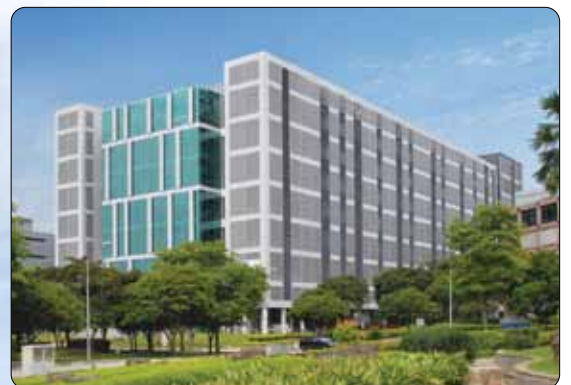
Jurong Data Centre 4,000 m 2
